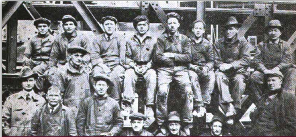
Members of Local 361 and sister Ironworkers locals 11, 30 and 45 erecting the Loew's State Theatre on 48th Street and Broadway in New York City in 1921.
