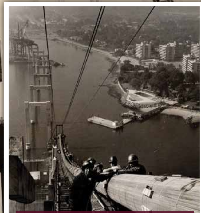
Local 361 members spin suspension cables through a saddle on top of a tower during construction of the Throgs Neck Bridge from October 1957 to its opening in January 1961.
